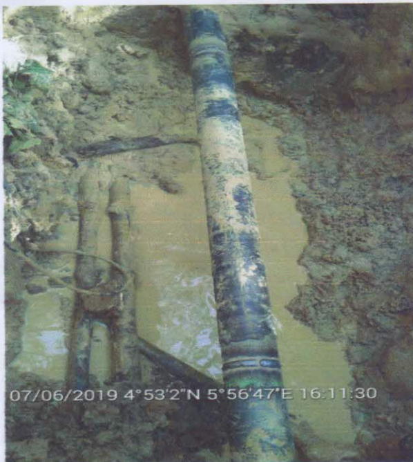
The bad section was cut-off and replaced.
